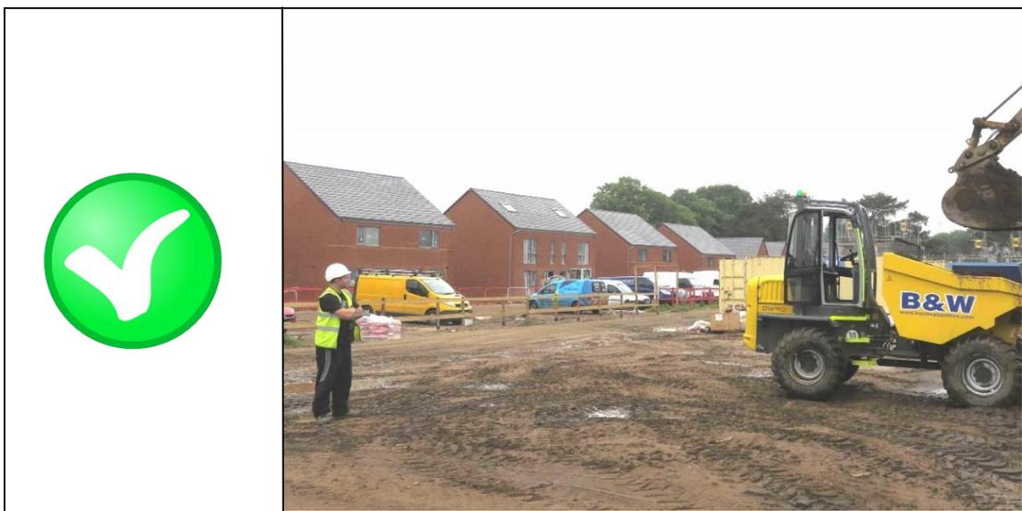
Figure 11 – Example of an operator clear of the loading activity
